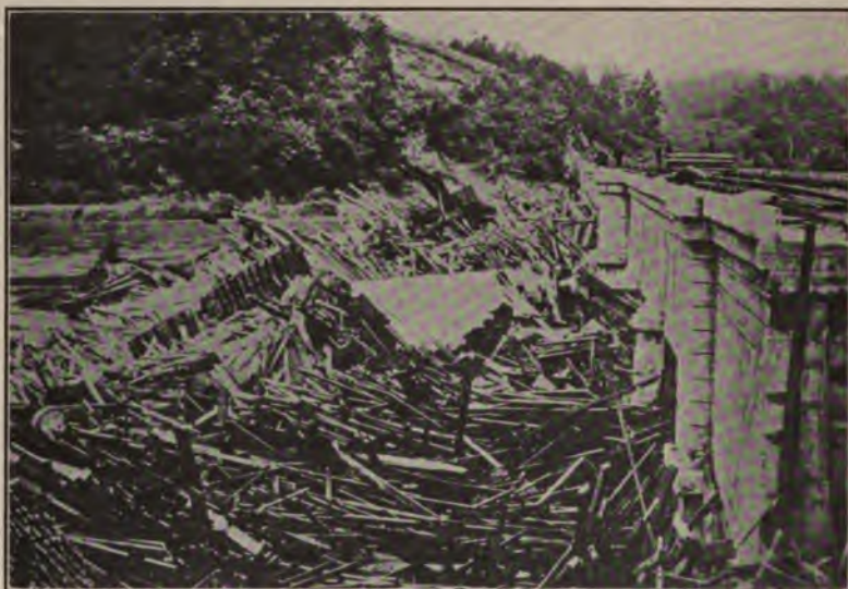
FIG. 29.—Flood debris above a viaduct. ( Courtesy of the Southern Railway. ) This illustrates the importance of a factor of safety in the design of openings and embankments.
